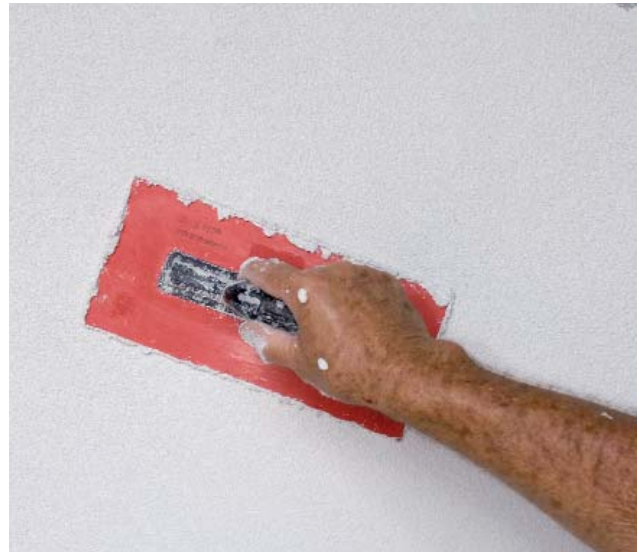
Application of Cemintel™ Texture Coat
